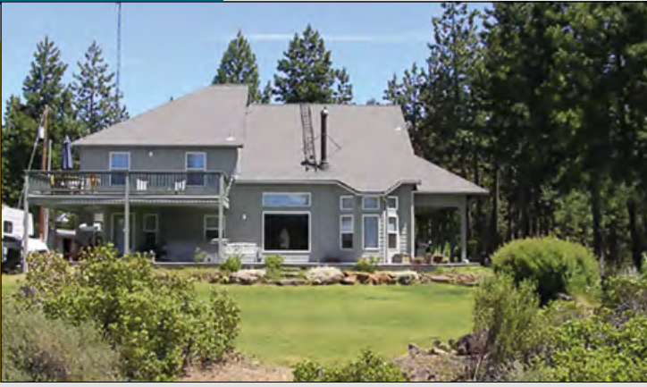
Figure 9. A well-maintained lawn can be part of a fire-wise landscape. Grass or alternative groundcovers serve as an effective fuel break. PHOTO: Stephen Fitzgerald, © Oregon State University
